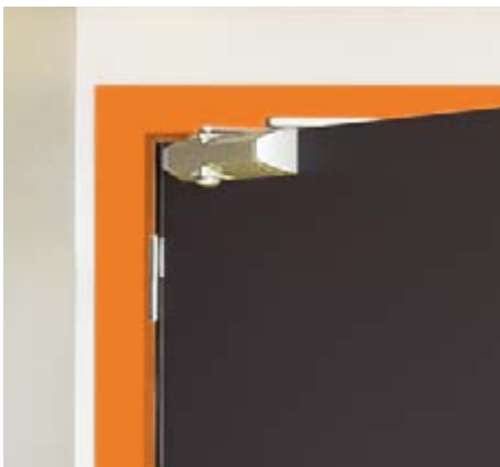
Door closer with scissor arm
